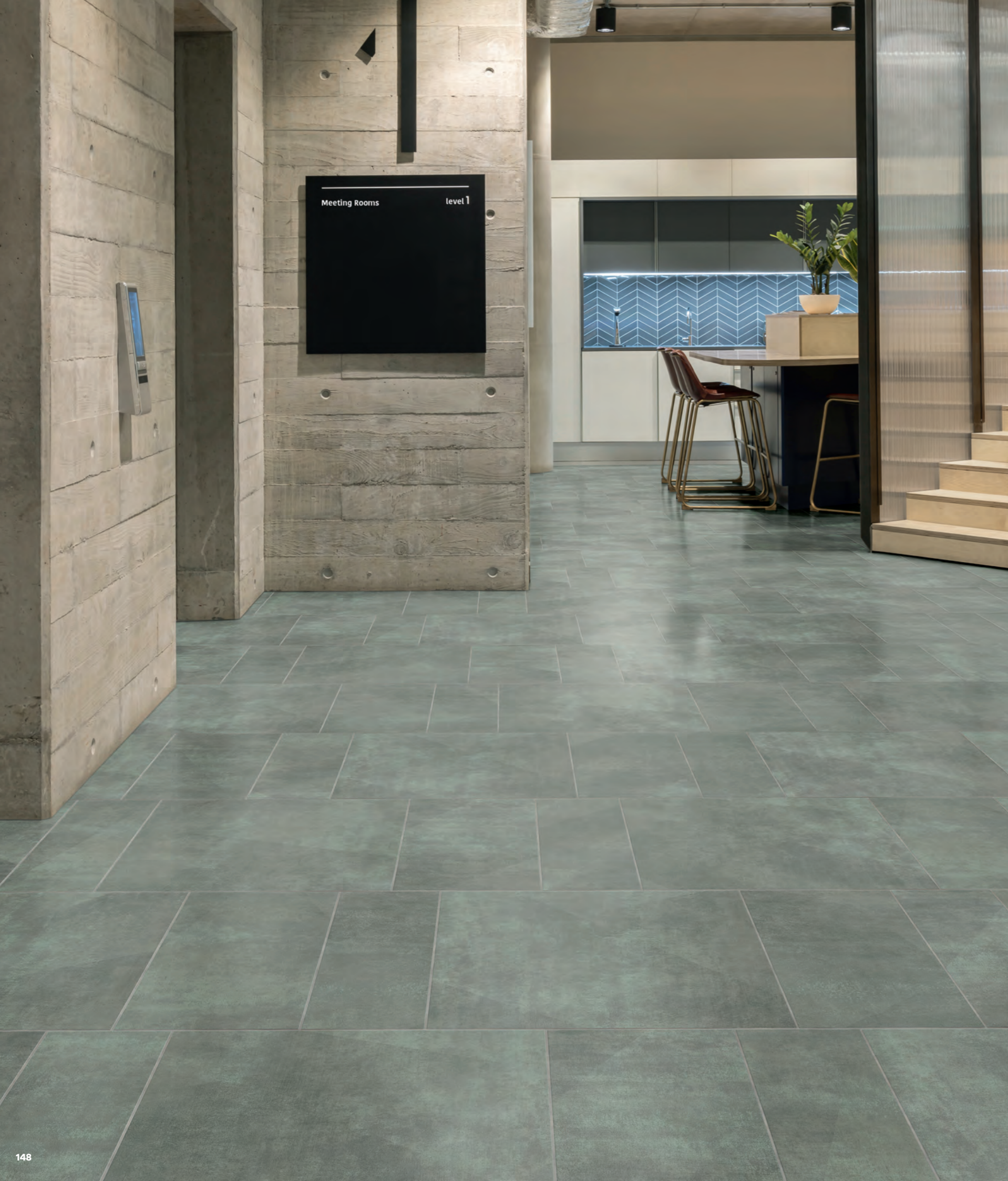
EP143 Staggered Block – Modernist Atrium & Modernist Spire Stripping
